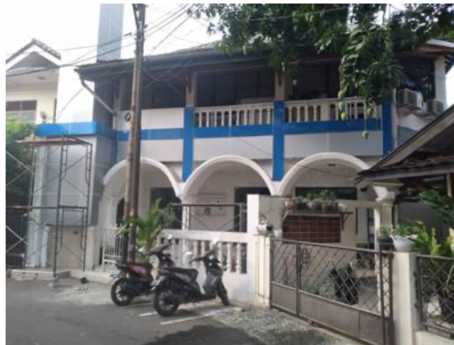
Gambar 13. Pekerjaan finishing facade.
