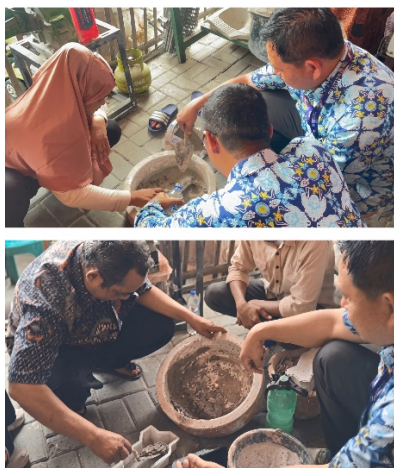
Figure 7. Paving block mixture making process
