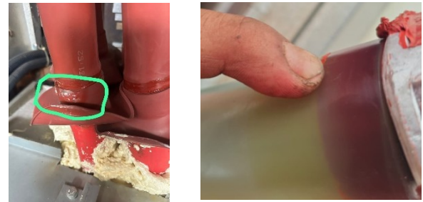
Fig 7 Visual Check Of Cable
