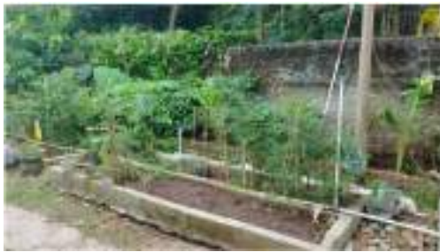
Figure 6. Installation of irrigation pipes
