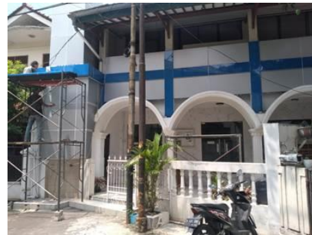
Gambar 13. Pekerjaan finishing facade.
