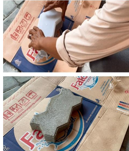
Figure 8. Paving Block Printing Process
